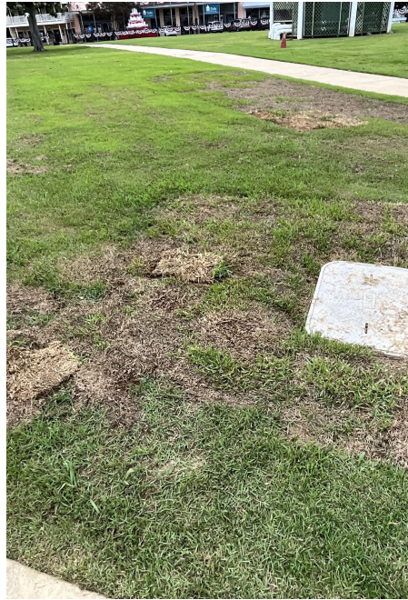
2 Sod to be replaced and holes sanded/filled.
