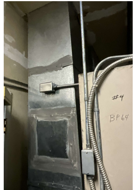
6 Completed mechanical duct work.
