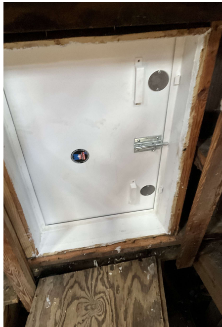
5 Completed roof door.
